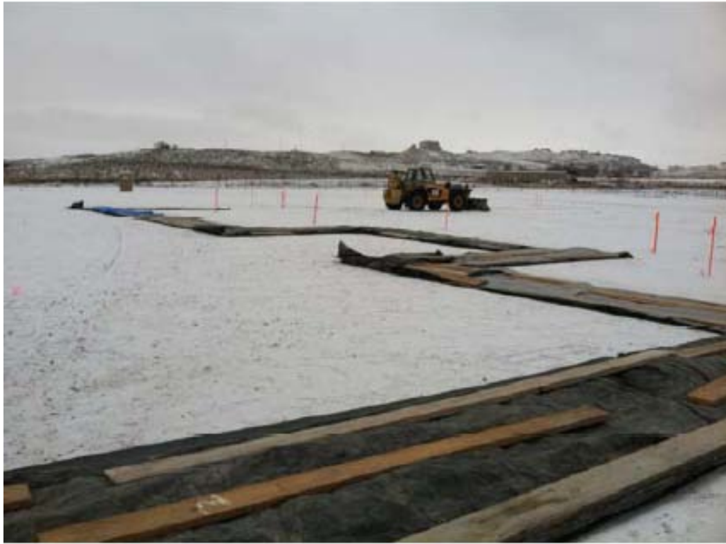
January 2014 - Ground thawing operation for building foundation
