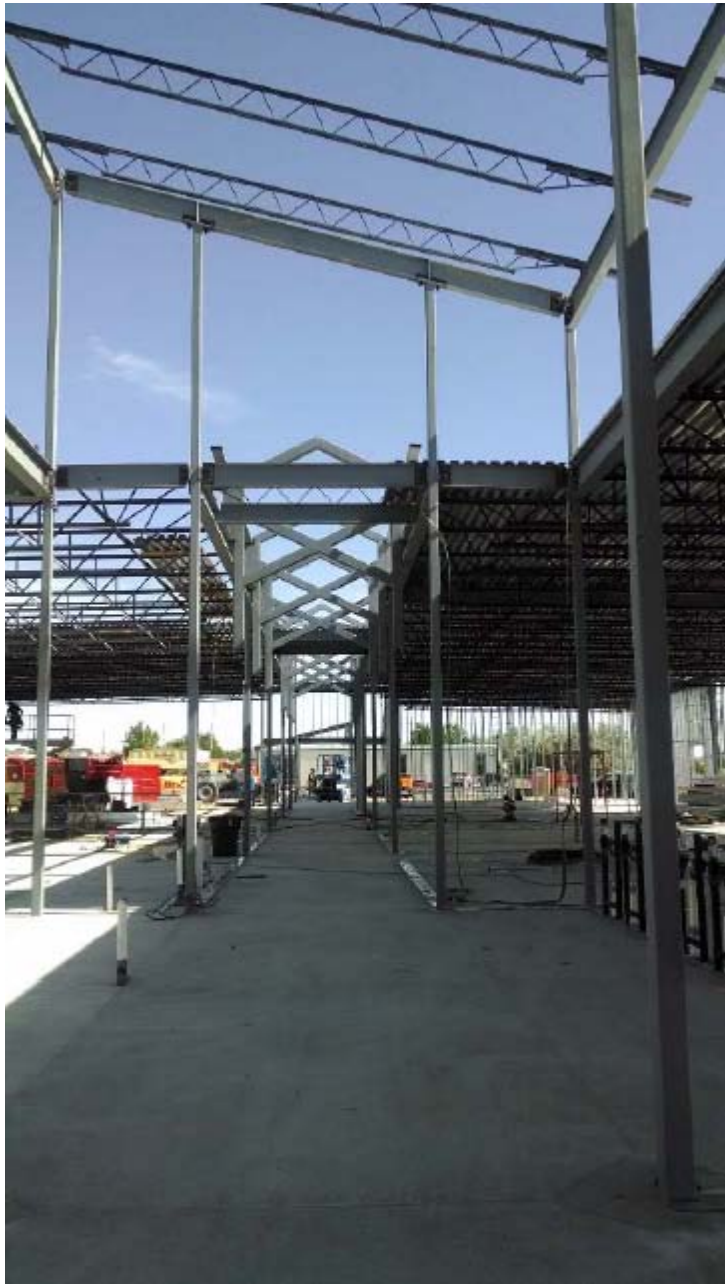
June 2014 – Building Interior taking shape
