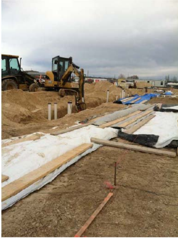
March 2014 – Underground Utility Construction
