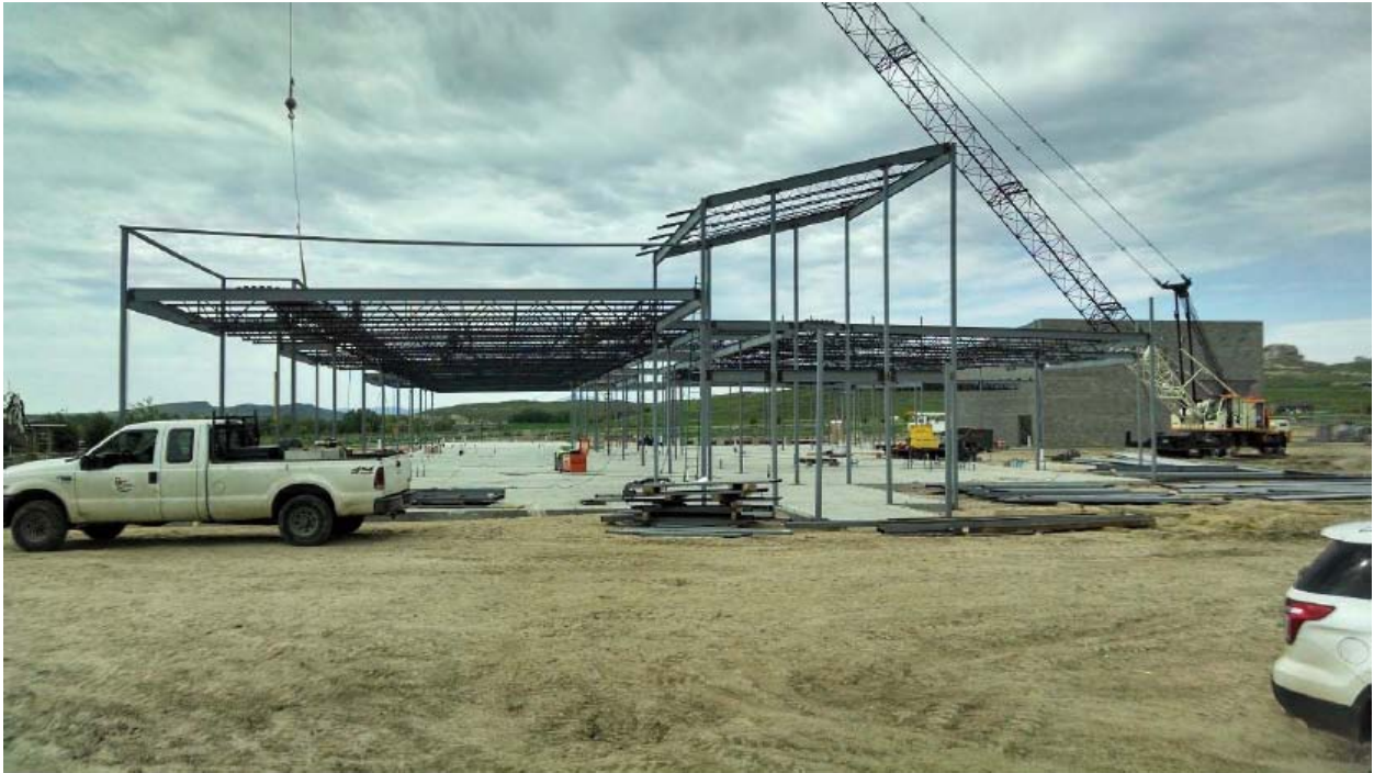
May 2014 – Structural Steel erection
