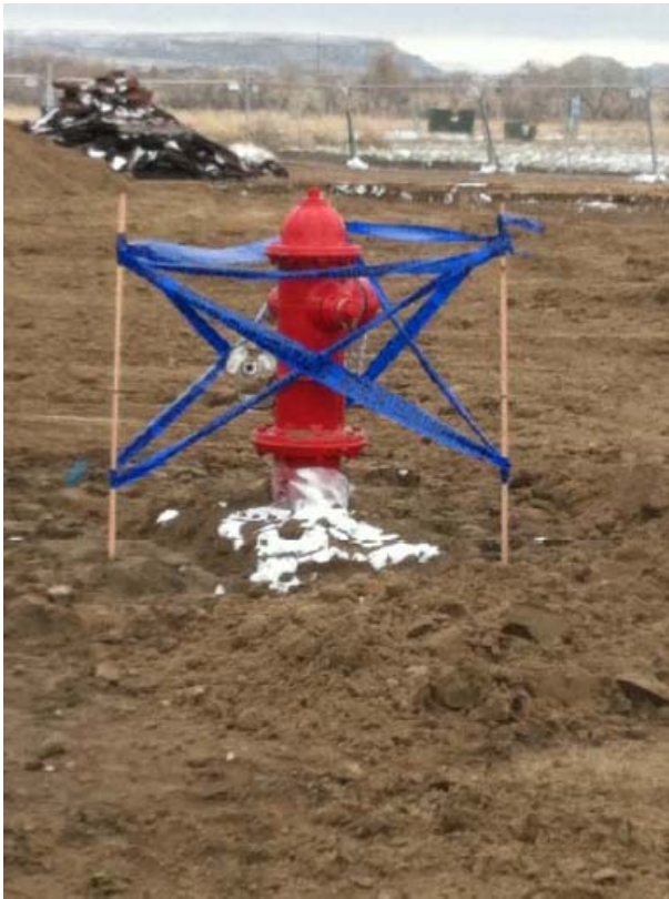
March 2014- Water System Installation
