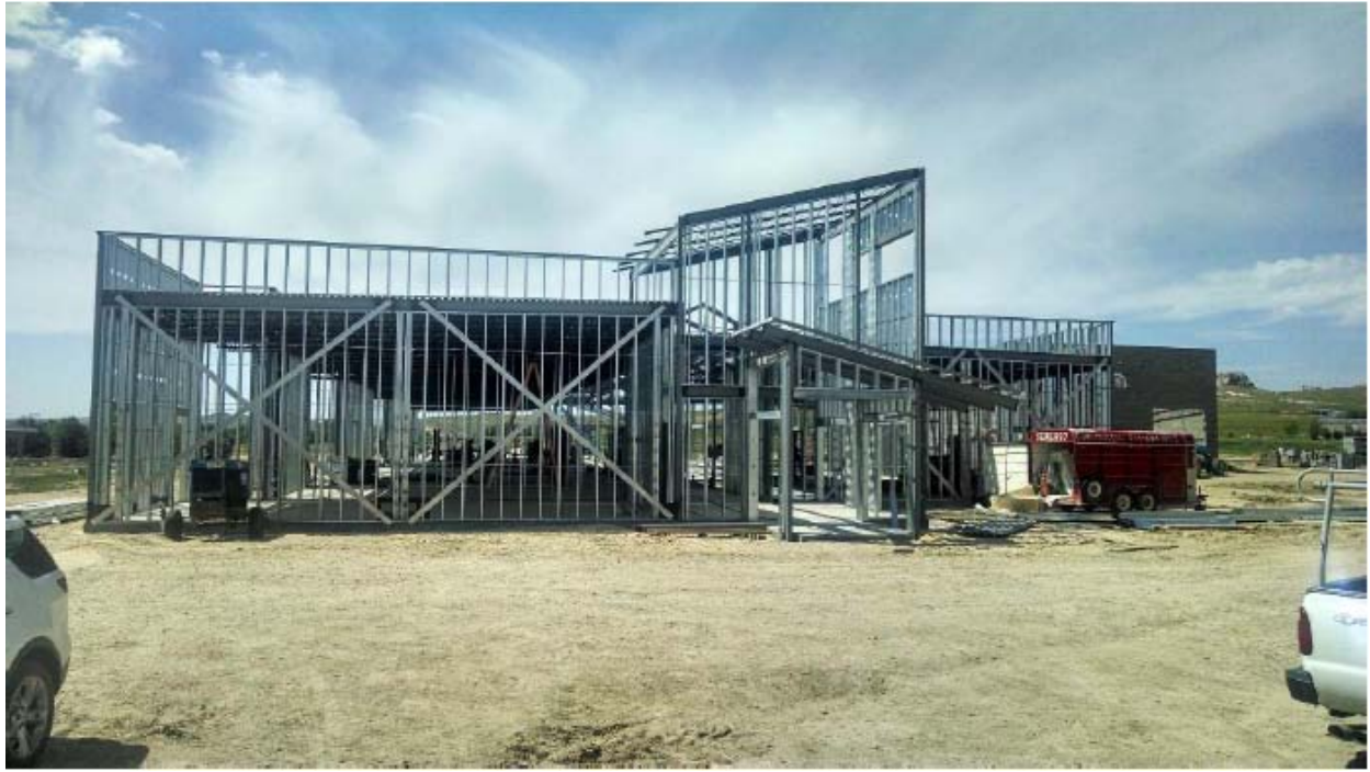
June 2014 – View of North Elevation
